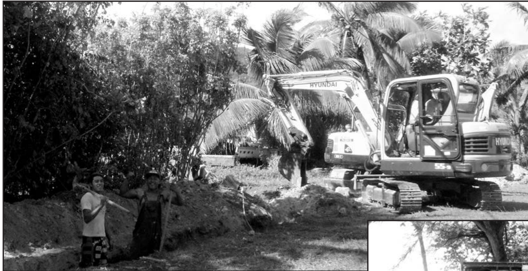
Right: Trenching for branch mains to homes off the main road near Turtles.
